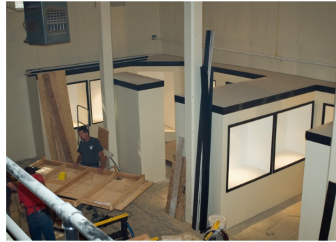
Before Demolition and Exhibit Cases Nearly Complete
